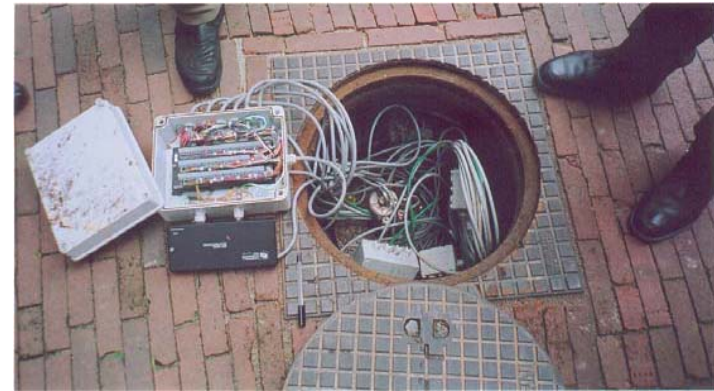
Real time extensometer & inclinometer installation
