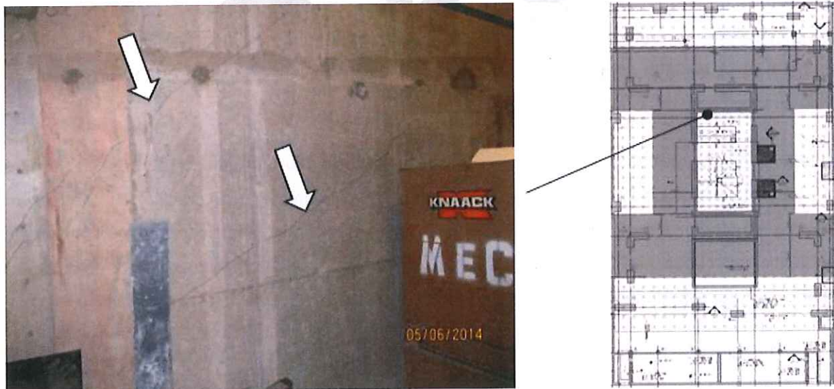
Figure 17 - Diagonal cracking shear wall adjacent to stair well
