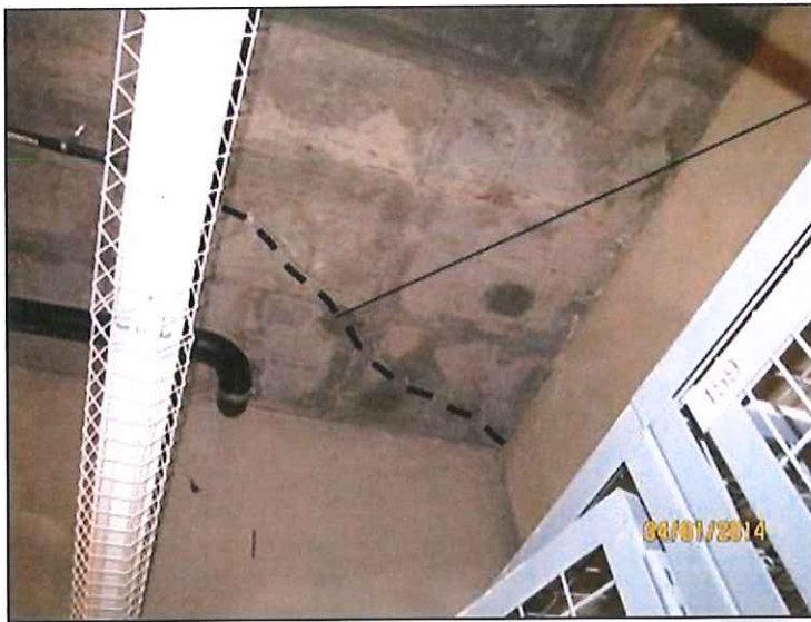
Figure 8 - Crack in underside of 1st floor slab
