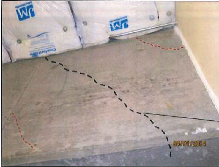
Figure 10 - Diagonal crack in moment frame beam, Line H near beam-column connection
