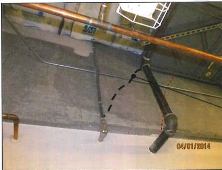
Figure 9 - Diagonal crack in moment frame beam along Line G.8 near beam-column joint
