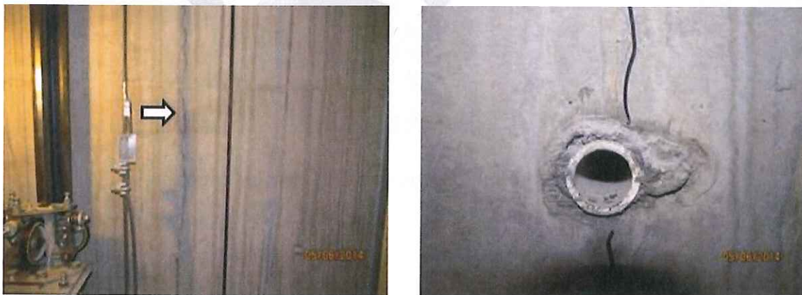
Figure 15 - Cracks observed in shear wall at elevator shift (a) from a distance and (b) at a penetration
